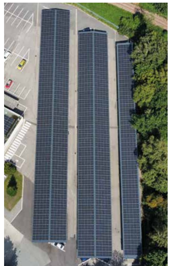
— PHOTOVOLTAIC SYSTEM on the employee car park: Shading and protection for cars
