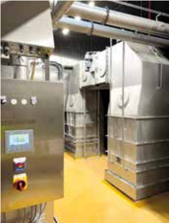
AIR RECIRCULATION of the CLIMAJet® KR-MAS systems
