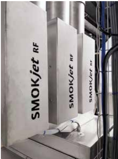
FRICTION SMOKE GENERATOR with 3-way outlet for alternating smoke supply
